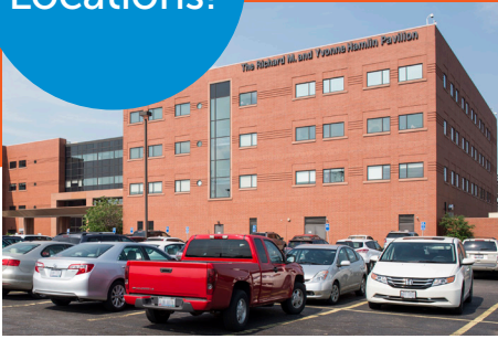
Summa Health System – Akron Campus, 95 Arch St, Suite 175, Akron, OH 44304
